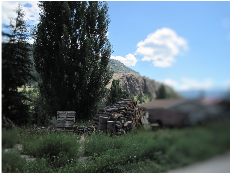
Figure 11 The presence of nearby vegetation and/or combustibles such as a woodpile that can ignite with relative ease and burn with high-intensity can present a hazard to a building's exterior. In this example, the woodpile has been situated far enough from the house so as to minimize this hazard.
