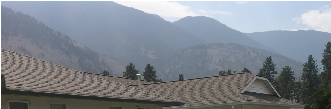
Figure 7 Roofs with a ULC rating, such as these asphalt composite shingles, provide a degree of fire resistance able to withstand ember ignition.
