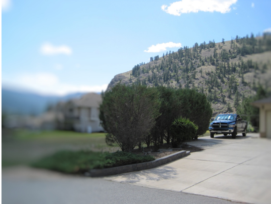
Figure 10 The cedar hedges pictured here have ladder fuels almost to the ground and have junipers beneath them. The junipers could ignite from embers and the trees could wick fire to the truck and subsequently ignite the house.
