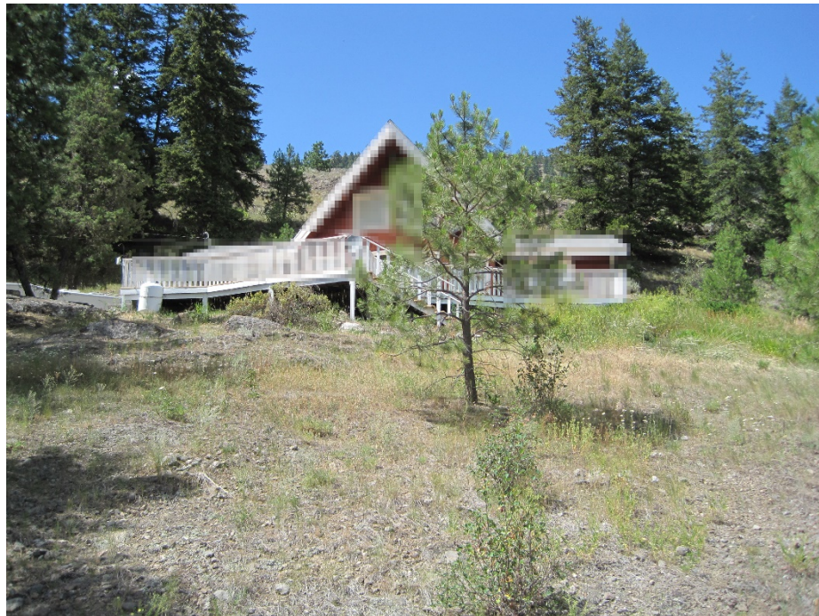
Figure 8 Decks that extend out over a slope require careful assessment of downslope fuels and the ignition potential of the deck.
