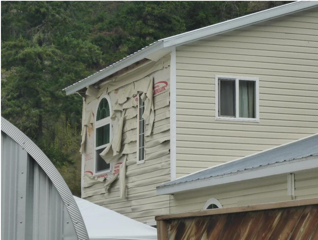
**Figure 11: Response of non-rated vinyl to melting during adjacent house fire.**
