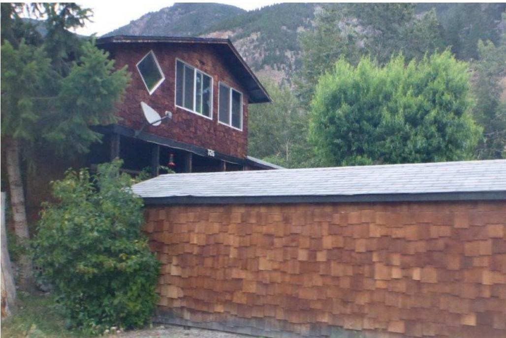
**Figure 10. Non-compliant homes with cedar shakes and wood cladding**
